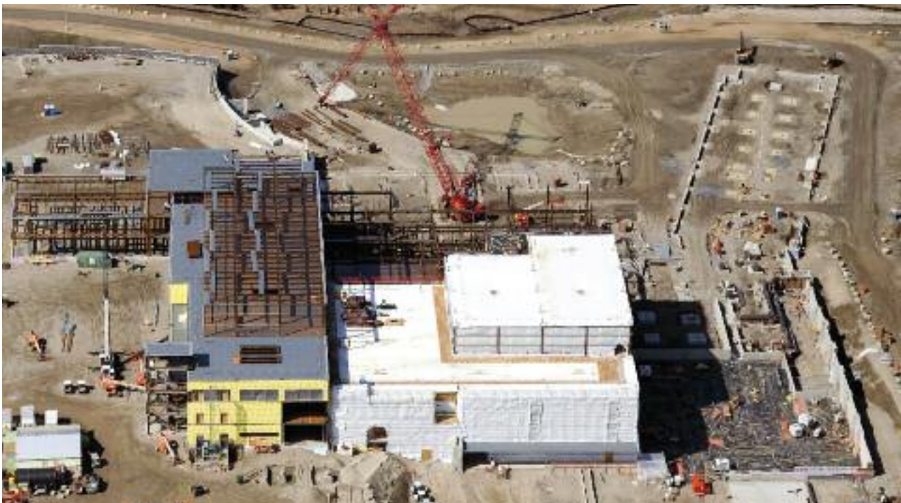
Figure 1. Aerial view of the hospital construction site
